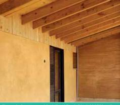
Figure 2: Compressed Stabilized Earth Block (CSEB) wall for Conservation Agriculture (RICA) Campus in Bugesera,
